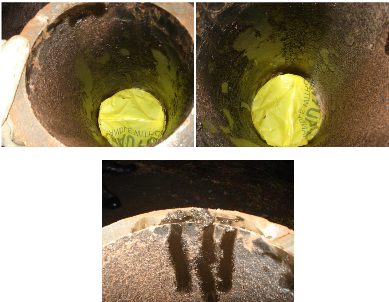
Figure 1: Pre-cleaning intervention pipe cut out
