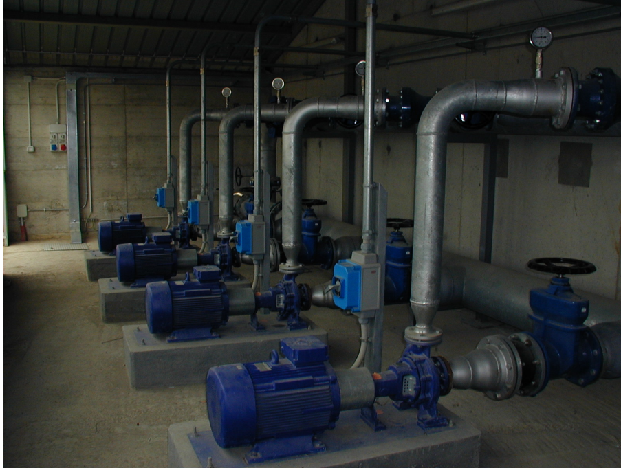
Fig. 1. A photograph taken inside the Casale pumping station, with the four pumps in parallel.
