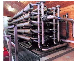
Fig. 1. Typical flow diagram and picture of a nanofiltration plant for NOM removal.
